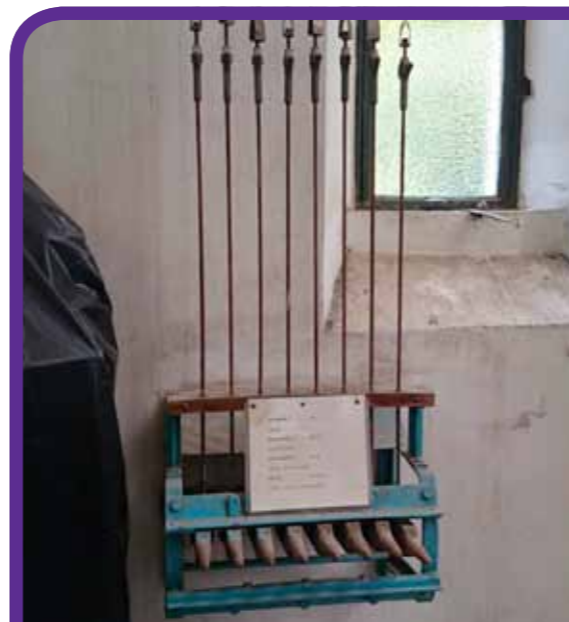
PHOTO 3 — The "Clavier" (keyboard) for manual ringing of the chime
